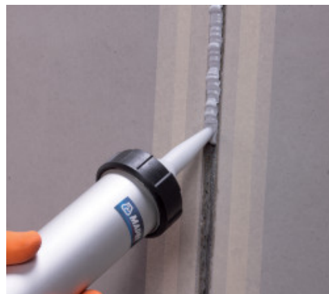
Application de Mapeflex PU40
